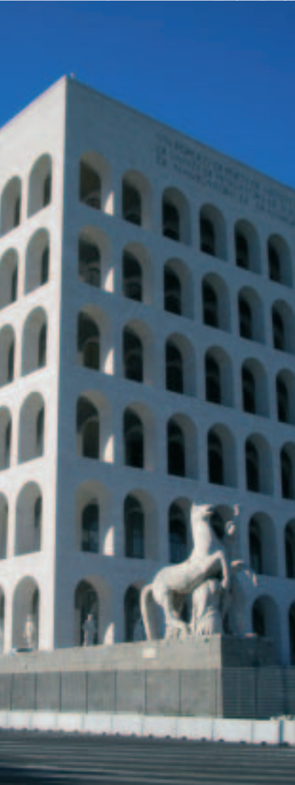
Palazzo della Civiltà Italiana (EUR-Rome). This building was cleaned, protected and consolidated with Kimia products.
