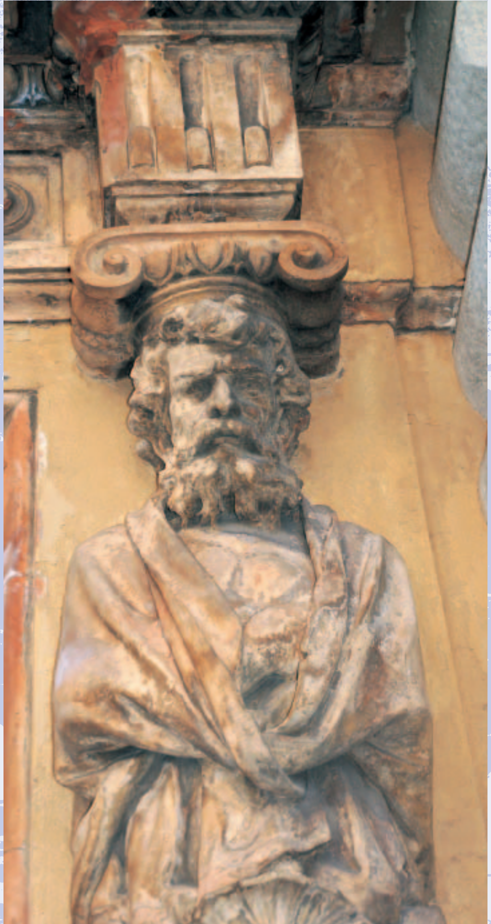
Atmospheric pollution triggers chemical processes that can alter the surface of natural stone materials used in historic buildings.
